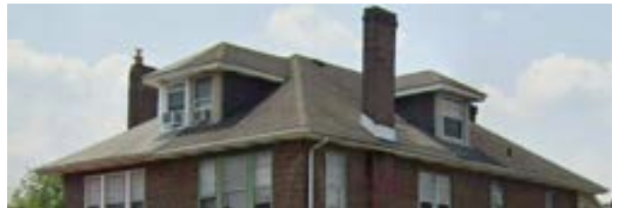
Pitched Roof Type (Hipped Roof)
