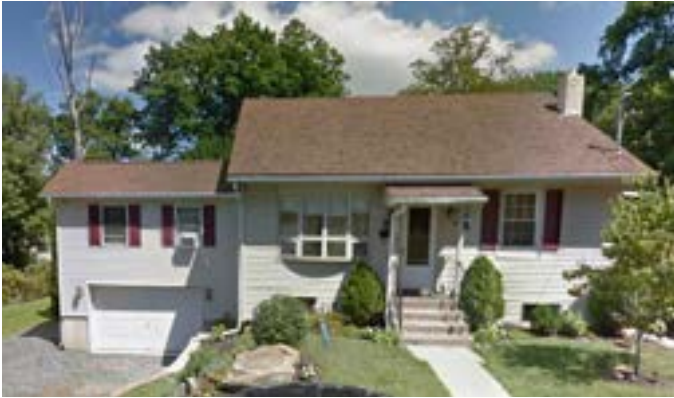
Figure 660-24(7) Full Height Basement Garage
