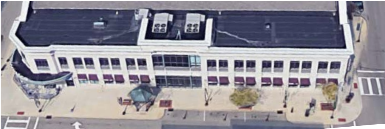
Figure 660(35) Rooftop Utilities Screened from the Public Way by a Parapet
