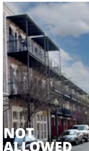
Balconies: Covers More than Allowed Facade Area
