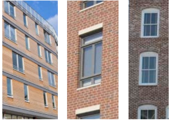
Figure 660(26) Vertically Oriented Windows with Expressed Lintels
