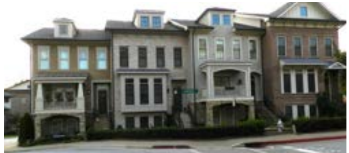
Stepped first floor levels with visible basements.
