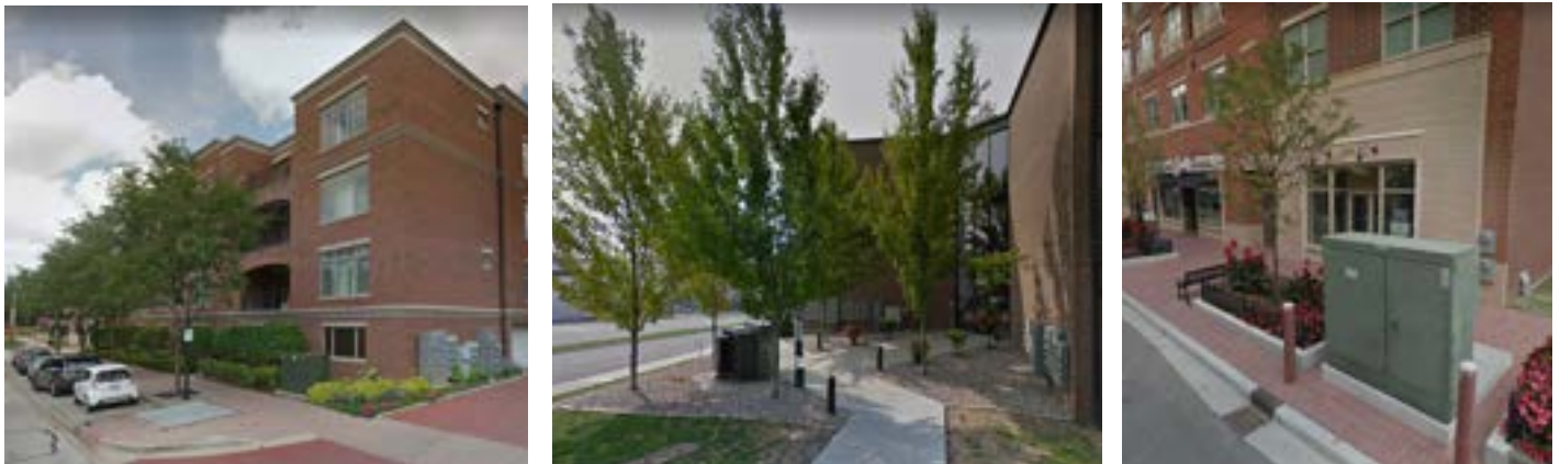
Figure 660(37) Examples of Poorly Located Utility Appurtenances on Front Streets
