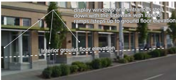
Figure 660(24) Storefront Windows Stepping with Sidewalk
